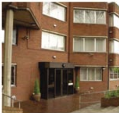
Prospect Point provides 38,424 sq ft. of quality office space TO LET a short walk from Gloucester city centre.
